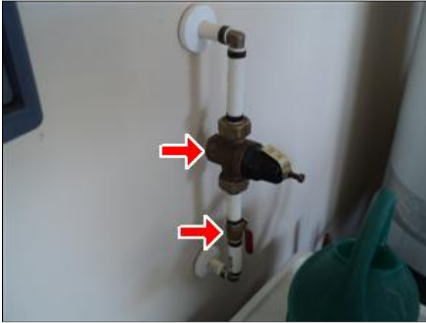
6.3 Picture 1 Interior cut off and regulator
