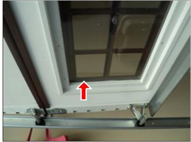
3.3 Picture 2 Garage window
